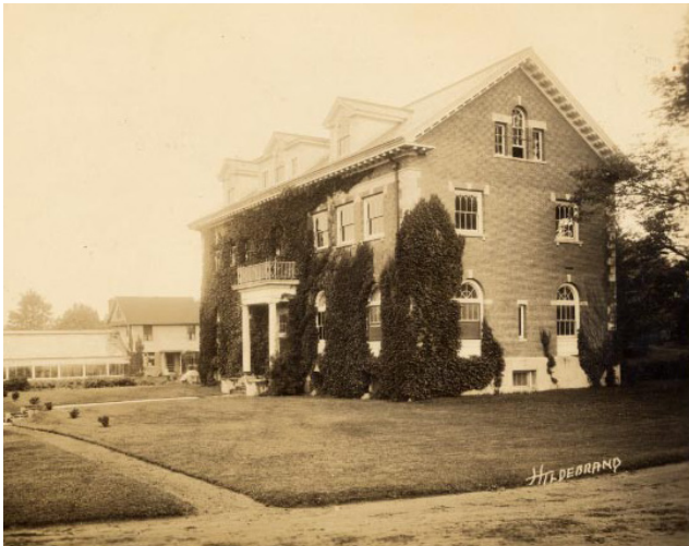
Note greenhouses next to the Budds Building, circa 1924.
